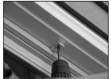
**2** – Grasp side rails and insert the bottom internal lock end caps. Next, insert both side rails onto protruding edge of housing end caps. Align rails plum into final position on window and fasten to window frame using screws.
